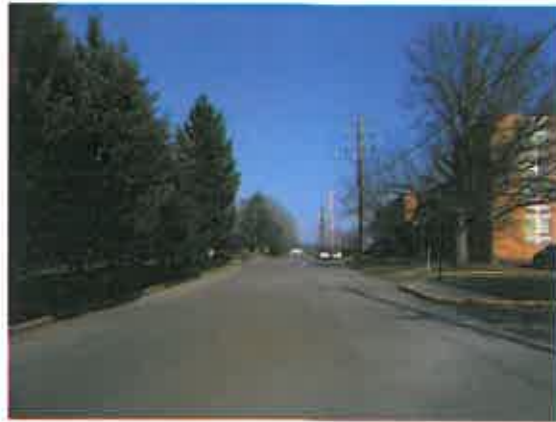
N. College Street at Carson-Newman College currently has sufficient pavement width to accommodate an on-road bicycle facility.
