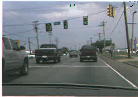
Major intersections along US 11 E (Andrew Johnson Highway) in Jefferson City, lack crosswalks and pedestrian signals near retail and commercial areas.
