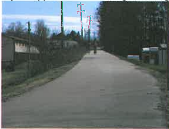
Abandoned railroad corridors provide connectivity to neighborhoods and parks in Jefferson City
