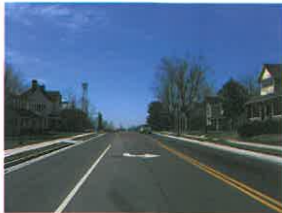
Sidewalks should be provided along both sides of residential streets that have lots less than one acre in size.
