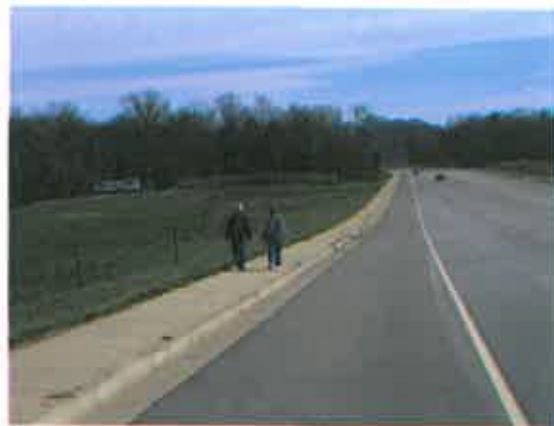
Pedestrians utilizing sidewalk along newly constructed SR 474 (Merchants Green Boulevard)
