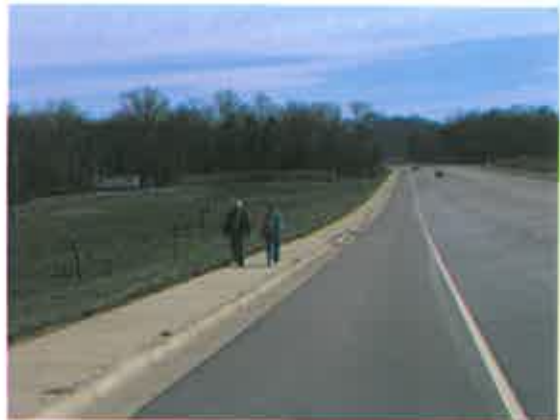
New and improved roadways should be designed as complete streets, providing accommodations for vehicles, bicycles, and pedestrians.
