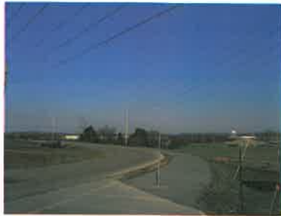
Greenway along Municipal Drive near Jefferson City Industrial Park
